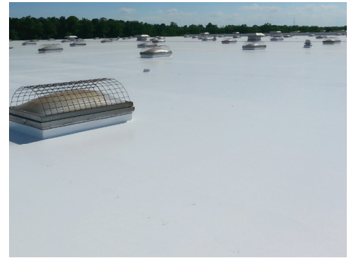
Reflective roof coating applied to a single-ply roof
