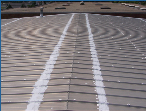
Metal roof with coating prep work completed at joints and fasteners
