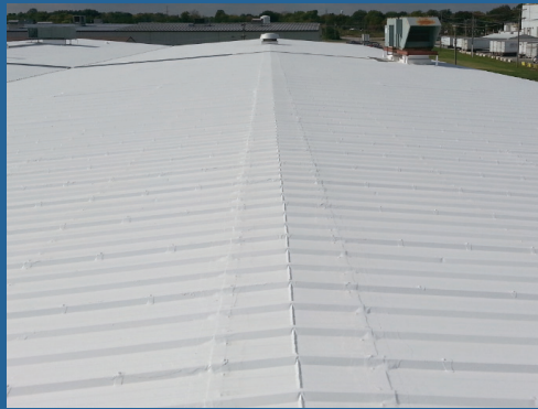
Reflective roof coating applied to a metal roof
